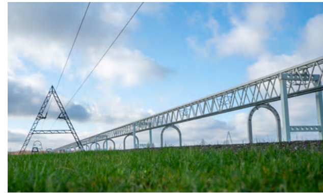
String Rail Overpass (track structure, intermediate supports and anchoring structures)
